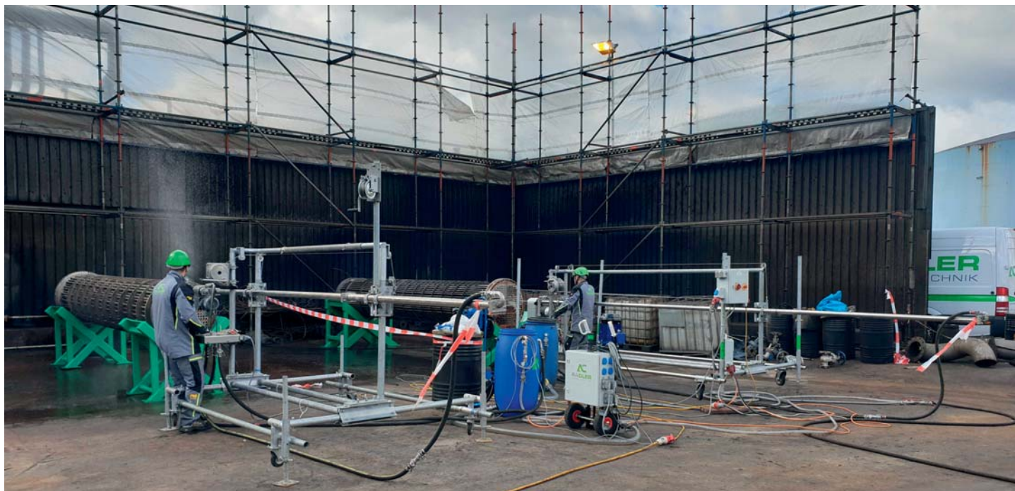
↗ Cleaning the tubes of two tube bundles with the RTC method.
